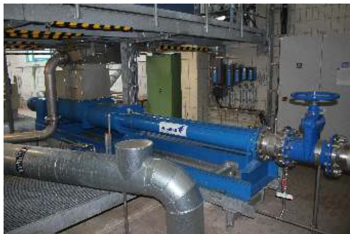
Four-stage solid-substance progressive cavity pump, type AE4N1450-RG from Allweiler®, used as residual sludge discharge pump, below the centrifuge.
