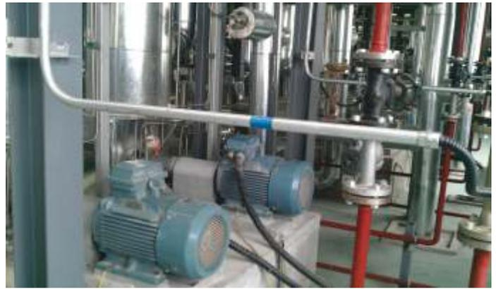
Pump, series CNH-B 32-250; liquid: T66 (Heat Transfer Oil)
