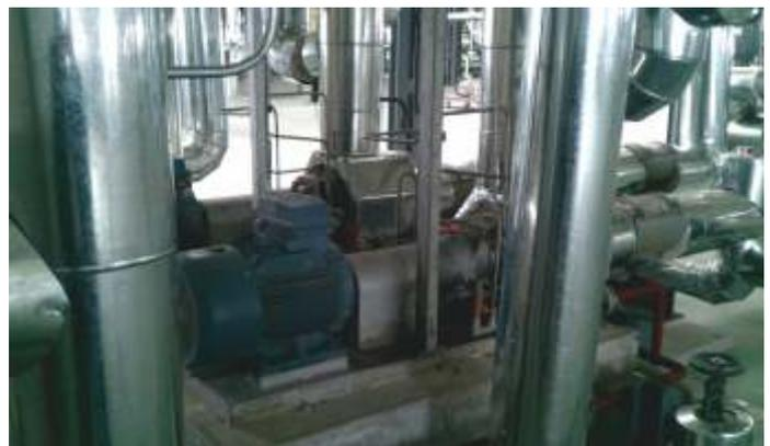
Pump series CNH-B 100-200; liquid: T66 (Heat Transfer Oil)
