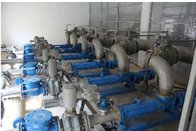
Application: Pump sludge Pump series: Tecflow 1001 Pressure: 4 bar (58 psi) Flow: 30 m 3 /h (132 gpm)
