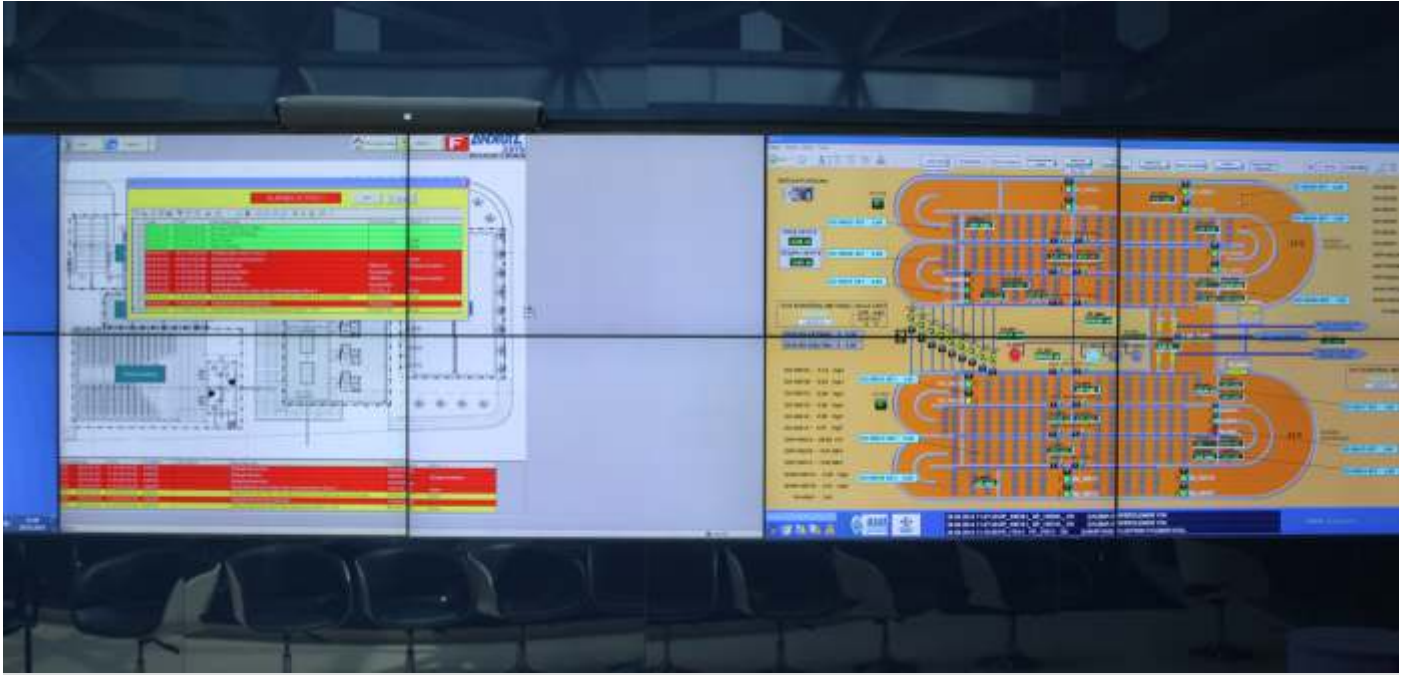
This plant's technology is unique in Turkey. Here it is shown on a video screen in a modern training room.
