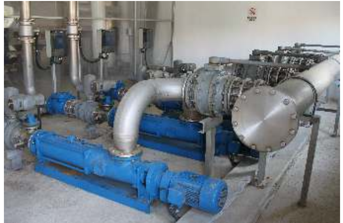
Application: Pump sludge Pump series: Tecflow 2701 Pressure: 1 bar (14.5 psi) Flow: 80 m 3 /h (352 gpm)
