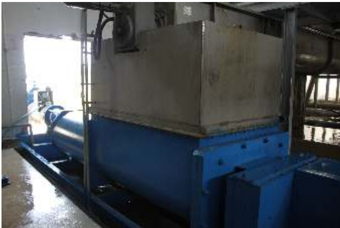
Application: Pump sludge for drying Pump series: Allweiler® AE 1+1N 5000-RG high-pressure progressing cavity pumps Pumping distance: 70 m (230 feet)
