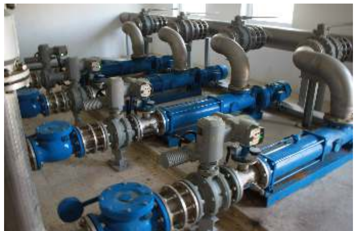
Application: Pump sludge Pump series: Tecflow 2701 Pressure: 1 bar (14.5 psi) Flow: 80 m 3 /h (352 gpm)
