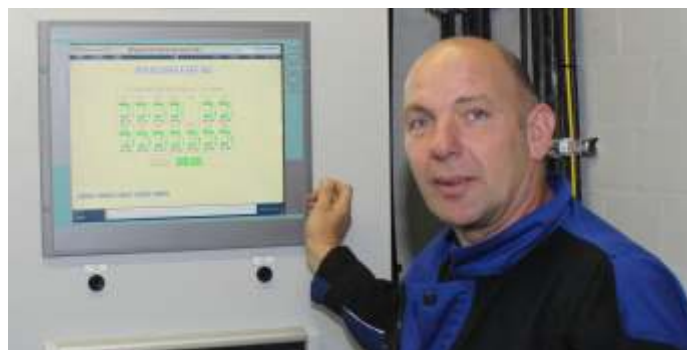
Falko Sellenk: "These pumps are extraordinarily reliable and need little maintenance."
