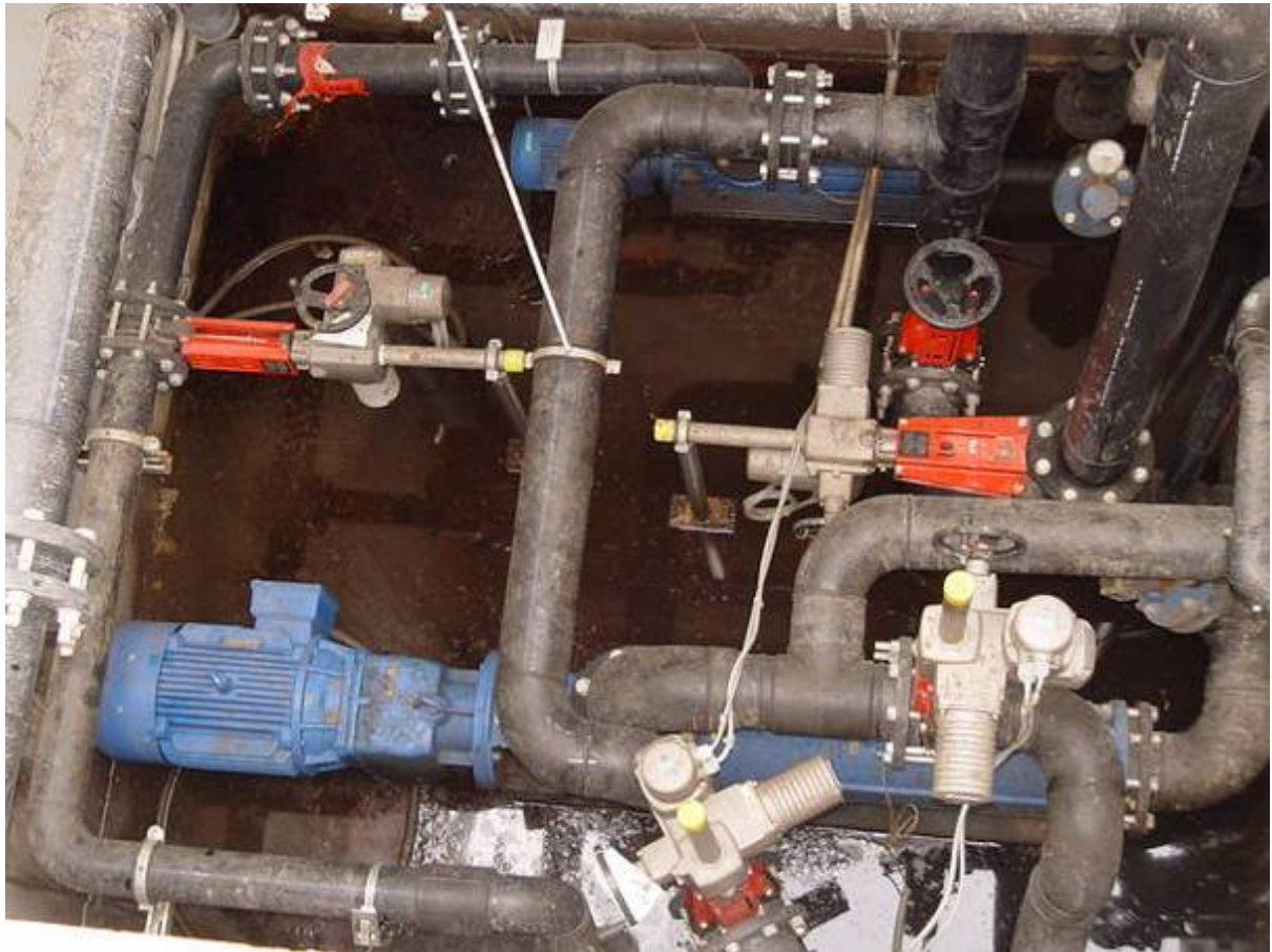
Allweiler progressing cavity pump of the AEB1E1450 series; liquid: digestates; capacity: 60 m 3 /hour; pressure: 4 to 5 bar.
