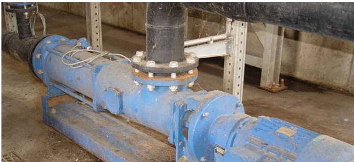
Allweiler progressing cavity pump of the AEB1E1450 series; liquid: process water; capacity: 60 m 3 /hour; pressure: 2 to 4 bar.
