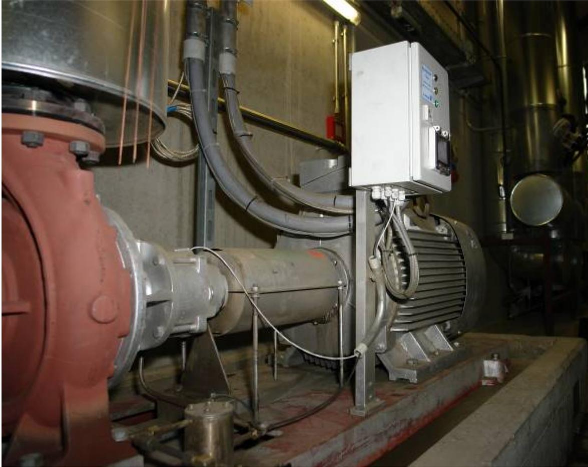
Allweiler Allheat thermal-oil pump with Allready Box (white device) in the biomass power plant. The cooperative makes any excess heat energy after the drying process available to local users. The pump moves thermal oil (Diphyl THT) at a pressure of 8.5 bar and a maximum flow rate of 285 m<sup>3</sup>/h.
