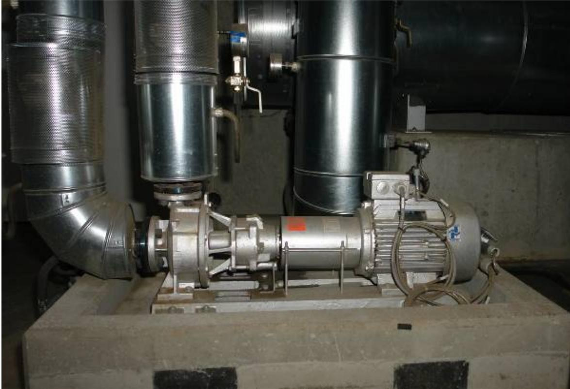
Allweiler pump of the Allheat series used as a circulation pump for emergency cooling. The liquid is a synthetic thermal oil (Diphyl THT), discharge pressure 3.5 bar, capacity 105 m<sup>3</sup>/h.
