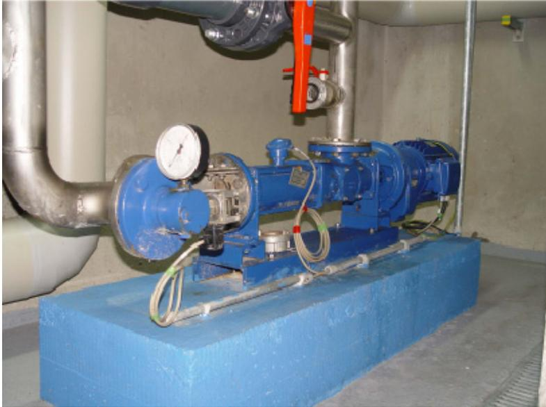
Feed pump of Allweiler's SEDBP series in size 300. Pumps fat to digestion tower (85 l/min).
