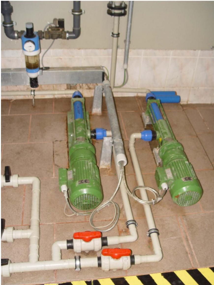
Allweiler progressing cavity pumps of the ANBP series used as flocculant pumps during drainage (max. 10 l/min at 12 bar and max. 20,000 mm<sup>2</sup>/s).
