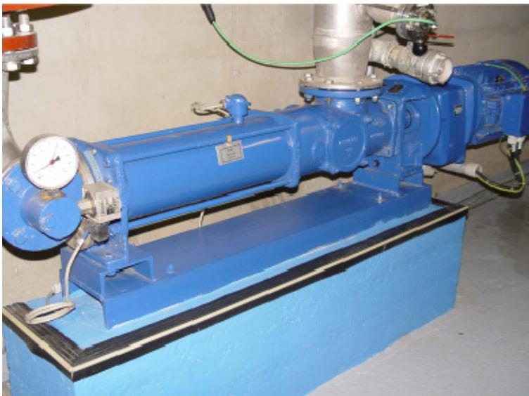
Pump SEBP 1000 for moving sludge to the primary sedimentation tank, capacity of 170 to 700 l/min.
