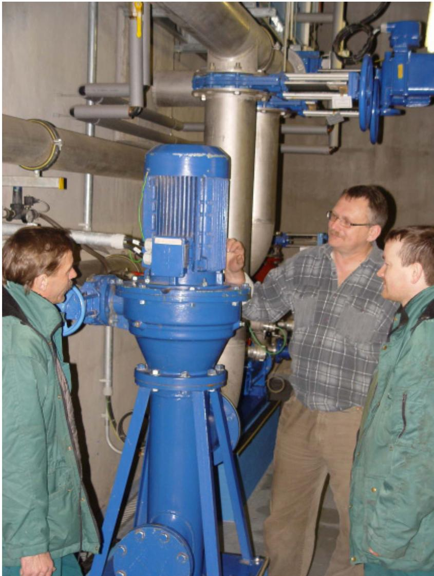
Macerator of type ABM 80-S in the primary-sludge feed line before primary sedimentation tank.
