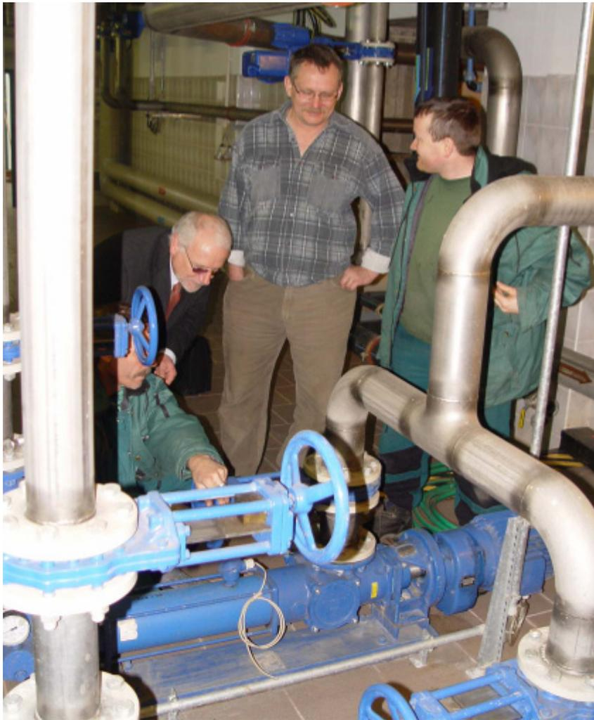
Progressing cavity pumps of the SEDBP 200 series for pumping fresh sludge to the digestion tower and centrifuges. Capacity of 170 l/min (max. 800 l/min, max. pressure 12 bar, viscosity up to 150,000 mm<sup>2</sup>/s).
