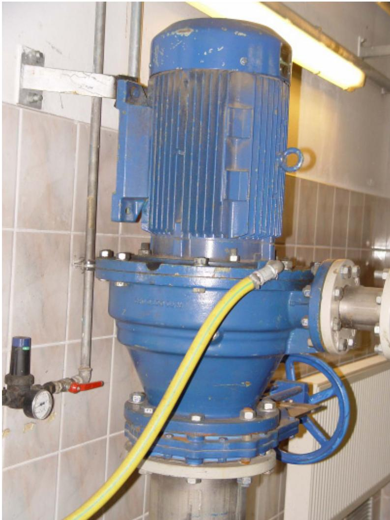
Macerator for feeding the digestion tower; ABM80-S series, capacity up to 160 m<sup>3</sup>/h.
