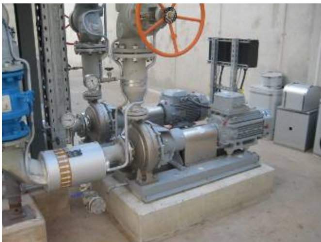
Centrifugal pump on working and pumping tanks for moving crude oil.
