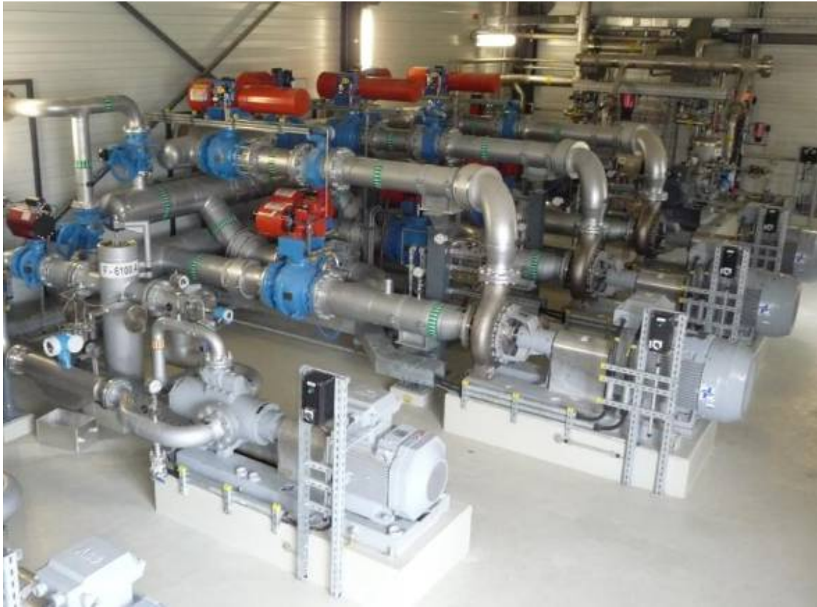
Allweiler pumps in the Matzen extraction station's pump house. In front a screw pump for pumping crude oil; behind that three centrifugal pumps for pumping formation water.
