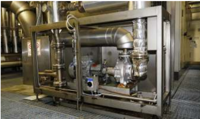
ALLHEAT® thermal oil pumps used at Alpenhain
