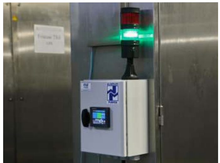
IN-1000 indicates normal operation of the monitored pumps.
