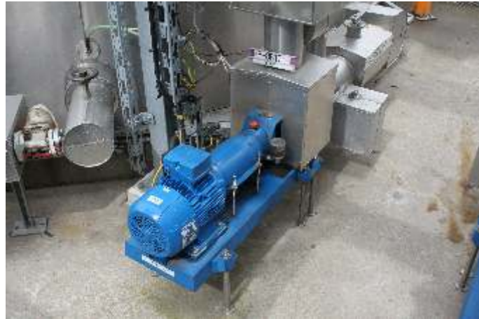
Series CNH-B 40-160/11 G-W20, capacity 20 m 3 /h, Liquid Farmin DM20, process: tank storage discharging.
