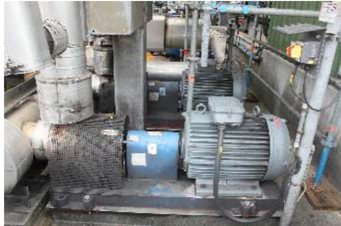
Alltherm series type CHT 65-250, capacity 75 m 3 /h, liquid thermal oil, process: heating system 250 °C.
