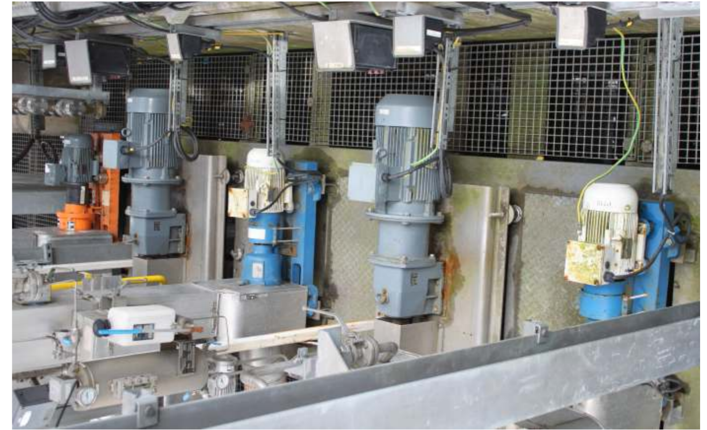
Series CMAL 32-200/1, capacity 15 m 3 /h, 1.2 bar, liquid caustic soda (50%), process: truck discharging. Series AK440-227-12, capacity 30 m 3 /h, 1 bar, 30 °C, liquid aqueous polycarboxylate, process: truck discharging. Series CMAL 32-200/1, capacity 15 m 3 /h, 0.9 bar, 40 °C, liquid phosphoric acid (75%), process: truck discharging. Series AK450-334-08, capacity 40 m 3 /h, 2.5 bar, 80 °C, liquid polyethylene glycol, process: truck discharging.
