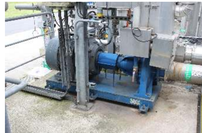
Series NT150-400/02, capacity 350 m 3 /h, 5 bar, liquid cooling water, process: cooling water system.
