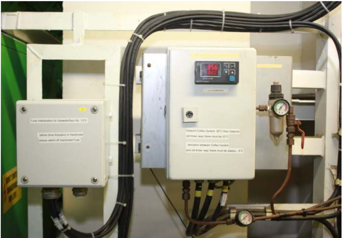
Wiring box (left) for the sensors of the CM-1000 system. Control box (right) for the controller drive of the three-way valve in the original controller of the LT cooling water system. On the Kyoto Express, its set point is always 4 °C below the set point of the CM-1000. This ensures that the "old" and "new" controllers do not mutually influence each other.
