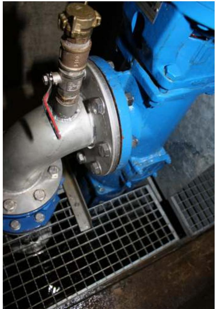
Colfax Fluid Handling Allweiler brand progressing cavity pump
