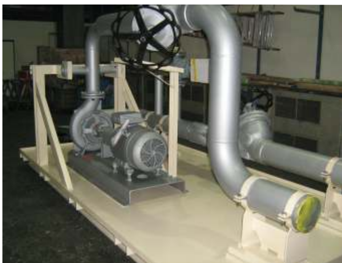
Secondary heating circuit with Allweiler® thermal oil pumps.
