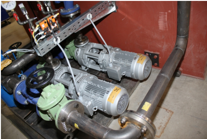
Two centrifugal pumps of the Allweiler® NBT series, circulating quenching oil.
