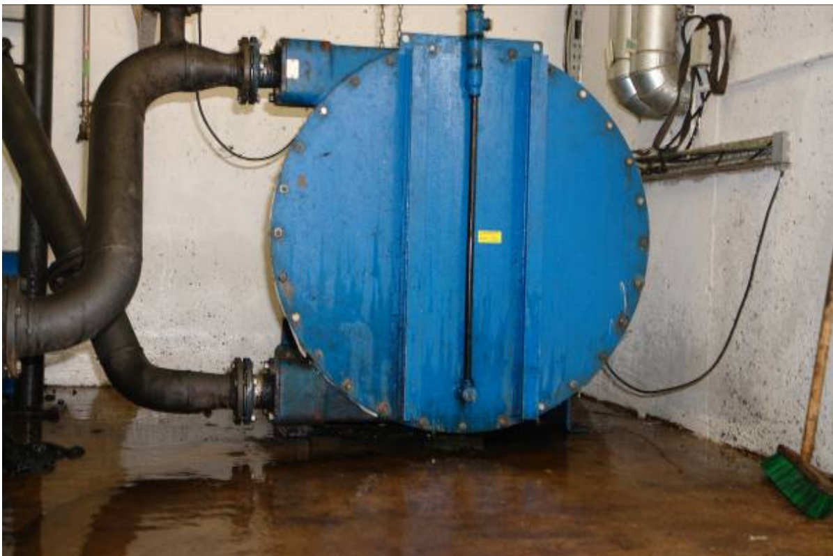
The most recent optimization (modified piping diameter) took place in the summer of 2006. Together with pressure and fill-level monitoring, hoses can now stay in service for up to 12 months.
