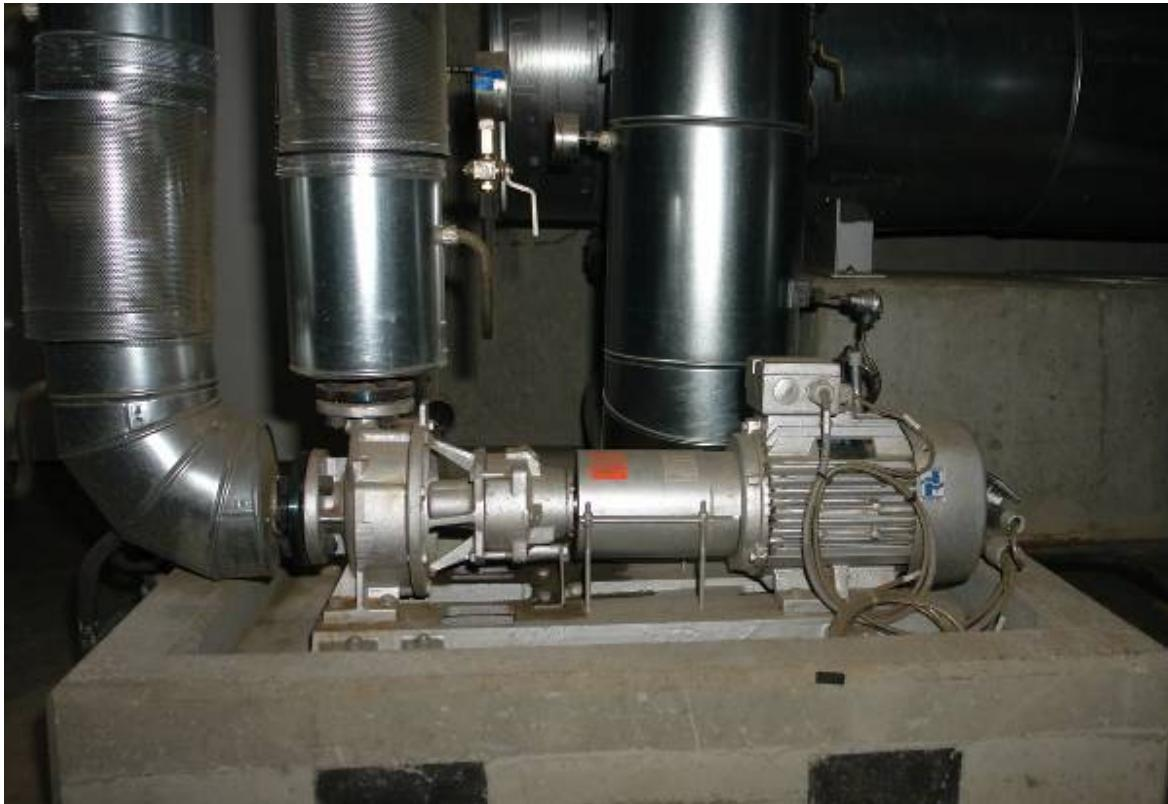
Allweiler pump of the Allheat series used as a circulation pump for emergency cooling. The liquid is a synthetic thermal oil (Diphenyl THT), discharge pressure 3.5 bar, capacity 105 m<sup>3</sup>/h.
