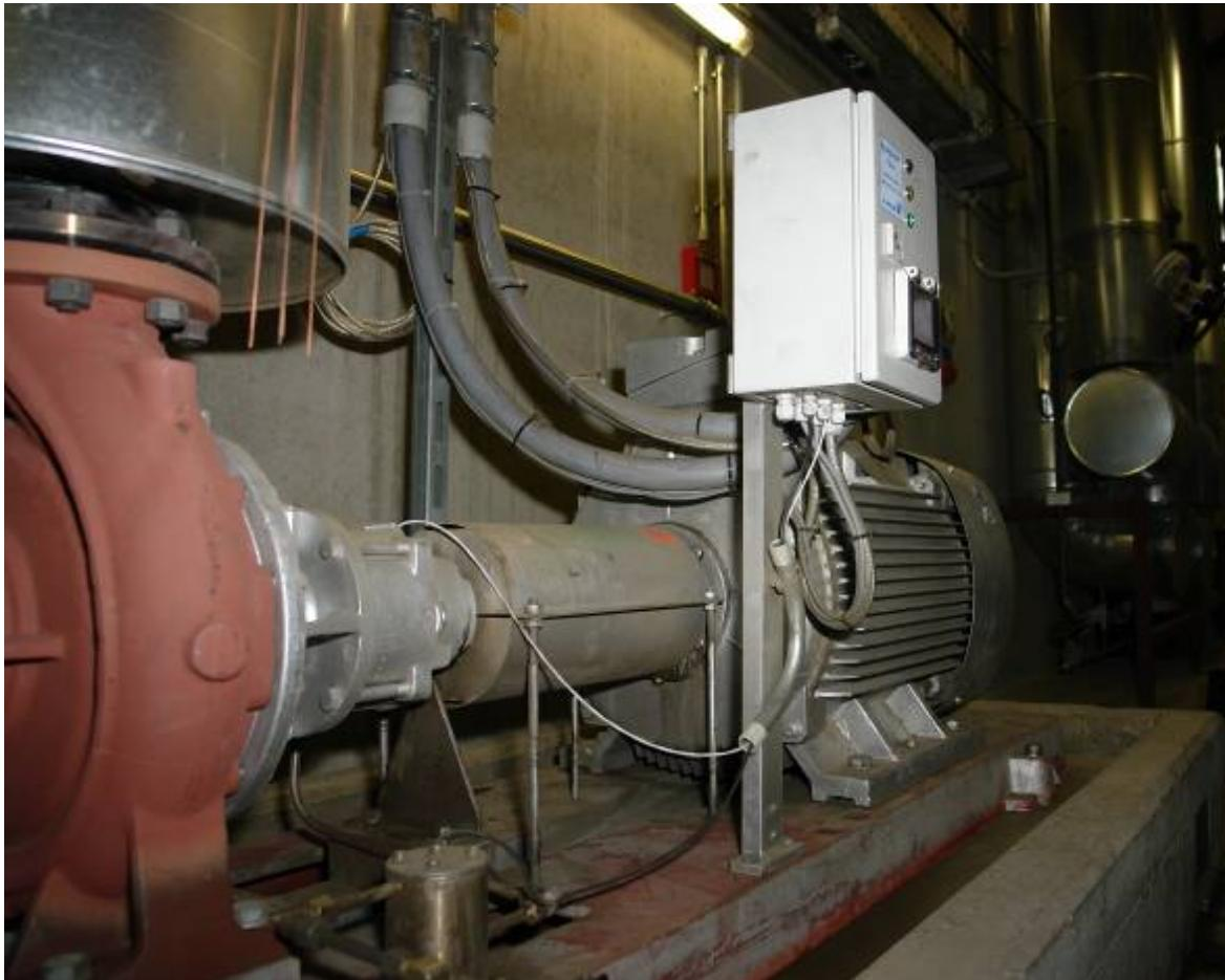
Allweiler Allheat thermal-oil pump with Allready Box (white device) in the biomass power plant. The cooperative makes any excess heat energy after the drying process available to local users. The pump moves thermal oil (Diphenyl THT) at a pressure of 8.5 bar and a maximum flow rate of 285 m<sup>3</sup>/h.
