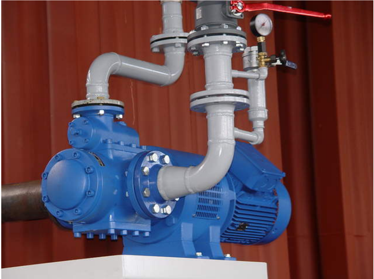
Screw pump of the "SN" series for moving base oils with viscosity of between 2 and 500 mm 2 /s. Capacity is about 200 l/min with discharge pressure of about 10 bar.
