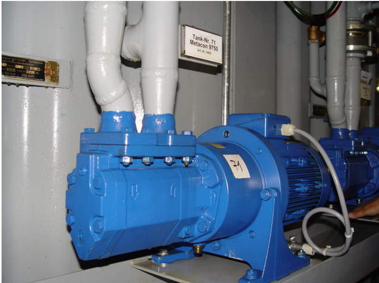
Screw pump for moving base oils like Metacon. Viscosity between 2 and 500 mm 2 /s. Capacity is about 150 l/min with discharge pressure of about 10 bar.
