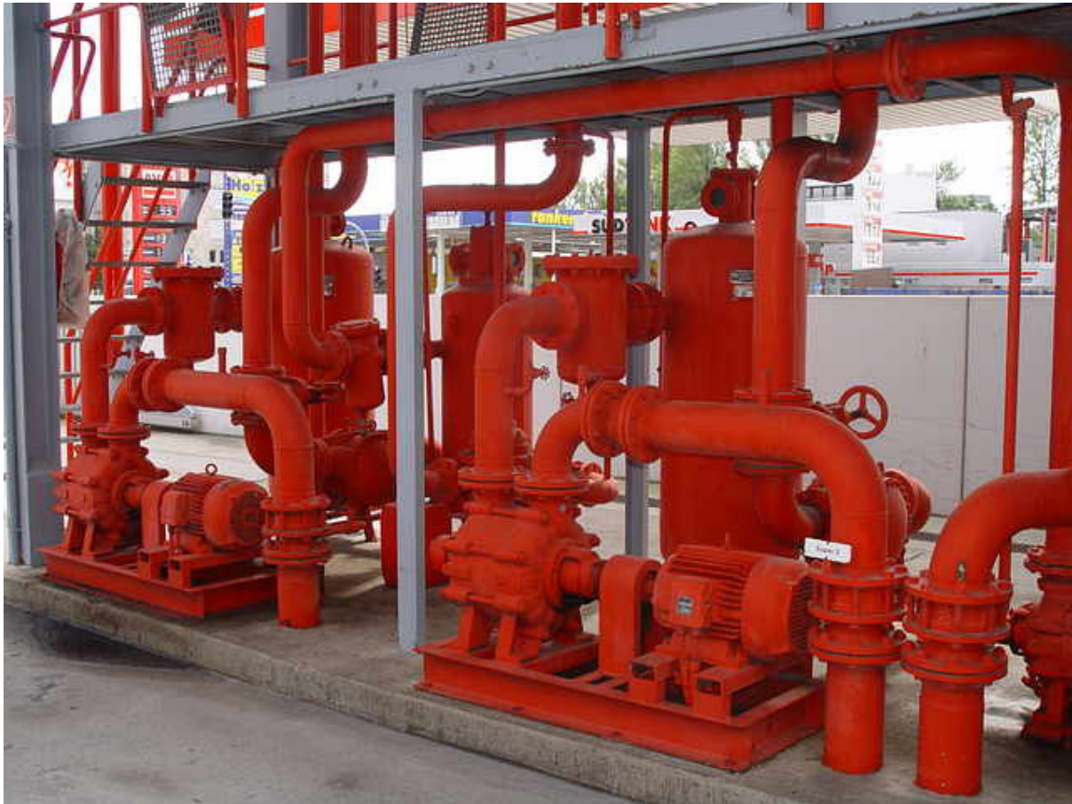
Filling plant for special-grade petroleum. Capacity of about 200 m 3 /h with delivery head of about 100 m.
