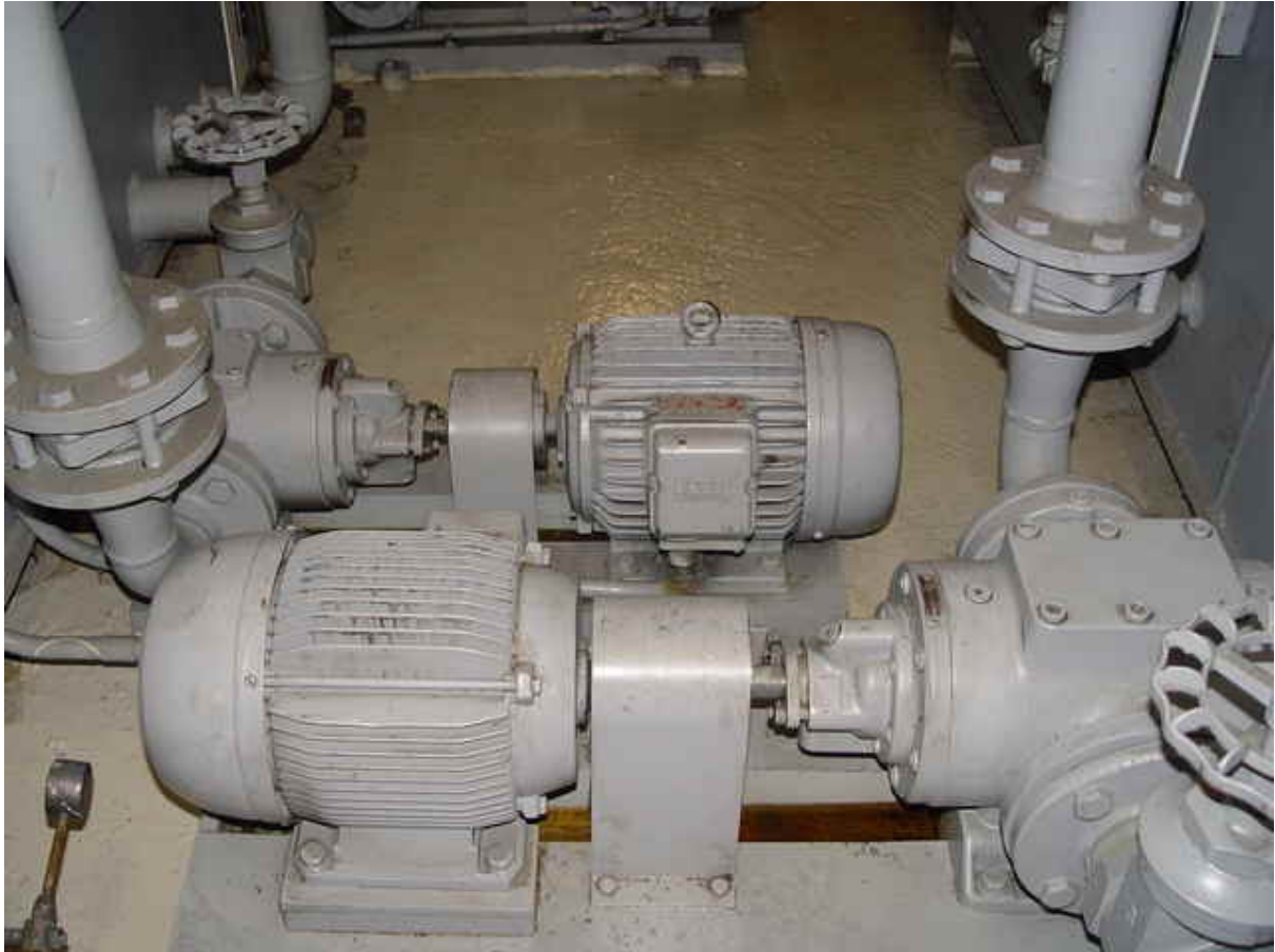
Two of about 40 screw pumps of the "SNH" series that have been moving base oils in the tank farm for about 30 years without failure or modification.
