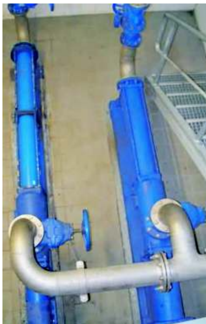
The AE..N preliminary filling pump for charging the chamber filter press (right) will be refurbished to make it identical to the existing AE..H (left).
