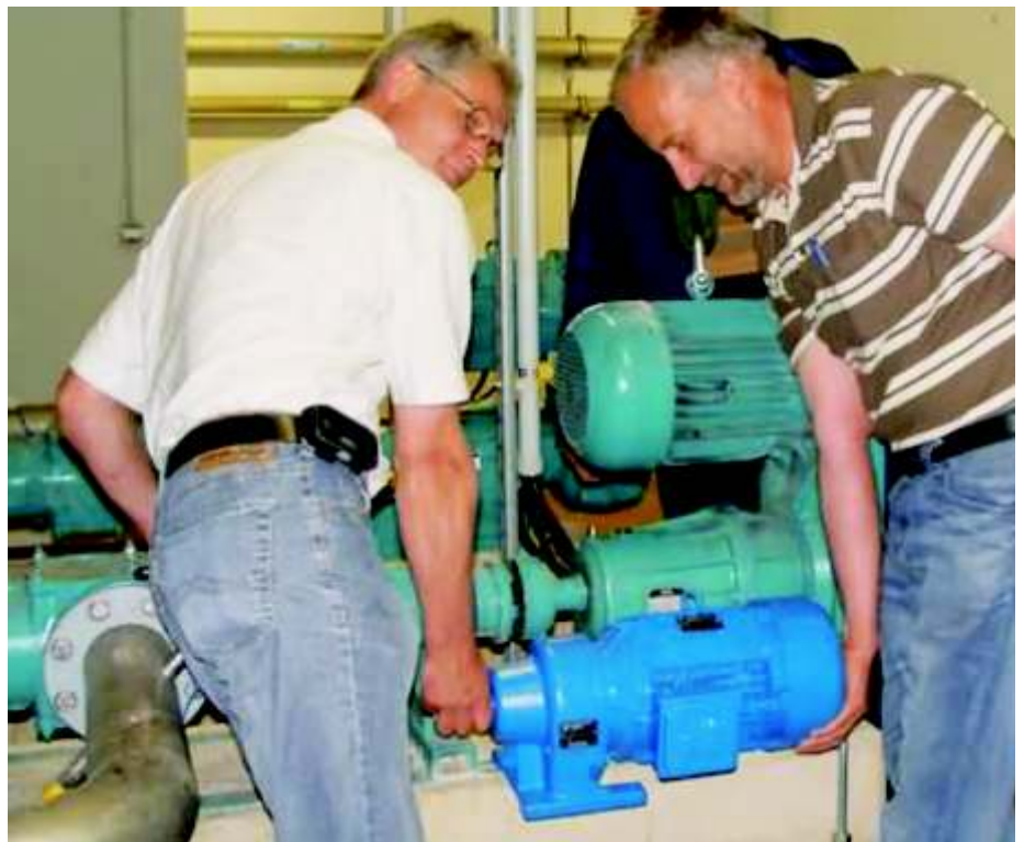
For comparison: The new, significantly smaller EFF1 motor is shown in front of the old belt-drive motor.
