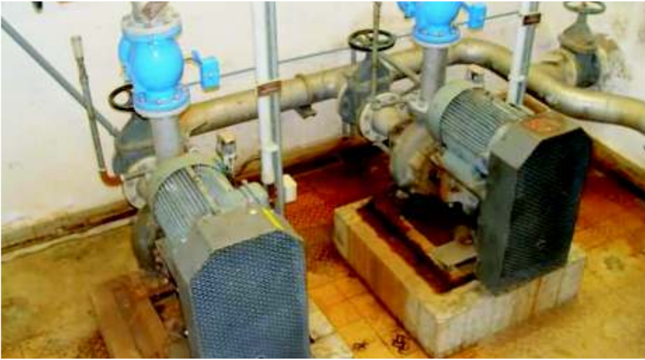
Allweiler's optimization recommendations made it possible to eliminate these two centrifugal pumps, saving the plant energy and maintenance costs.
