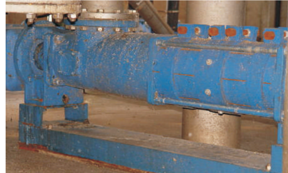
ALLWEILER progressing cavity pump of the AEB1E2700 series, with readjustable stator; medium: biomass; capacity: 100 m 3 /hour; pressure: 2 bar.
