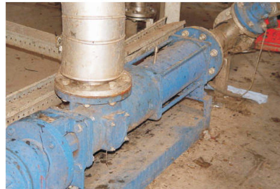
ALLWEILER progressing cavity pump of the AEB1E750 series; liquid: biomass at 75 °C; capacity: 18 m 3 /hour; pressure: 2-4 bar.
