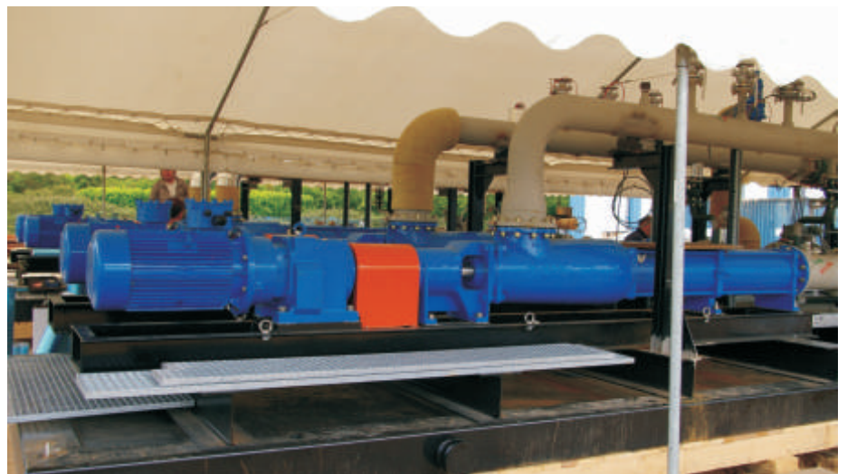
ALLWEILER dehydrator/desalter and heat exchanger feeding progressing cavity pumps.
